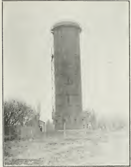
WORKING IN AN AWKWARD POSITION ON A WATER TOWER
